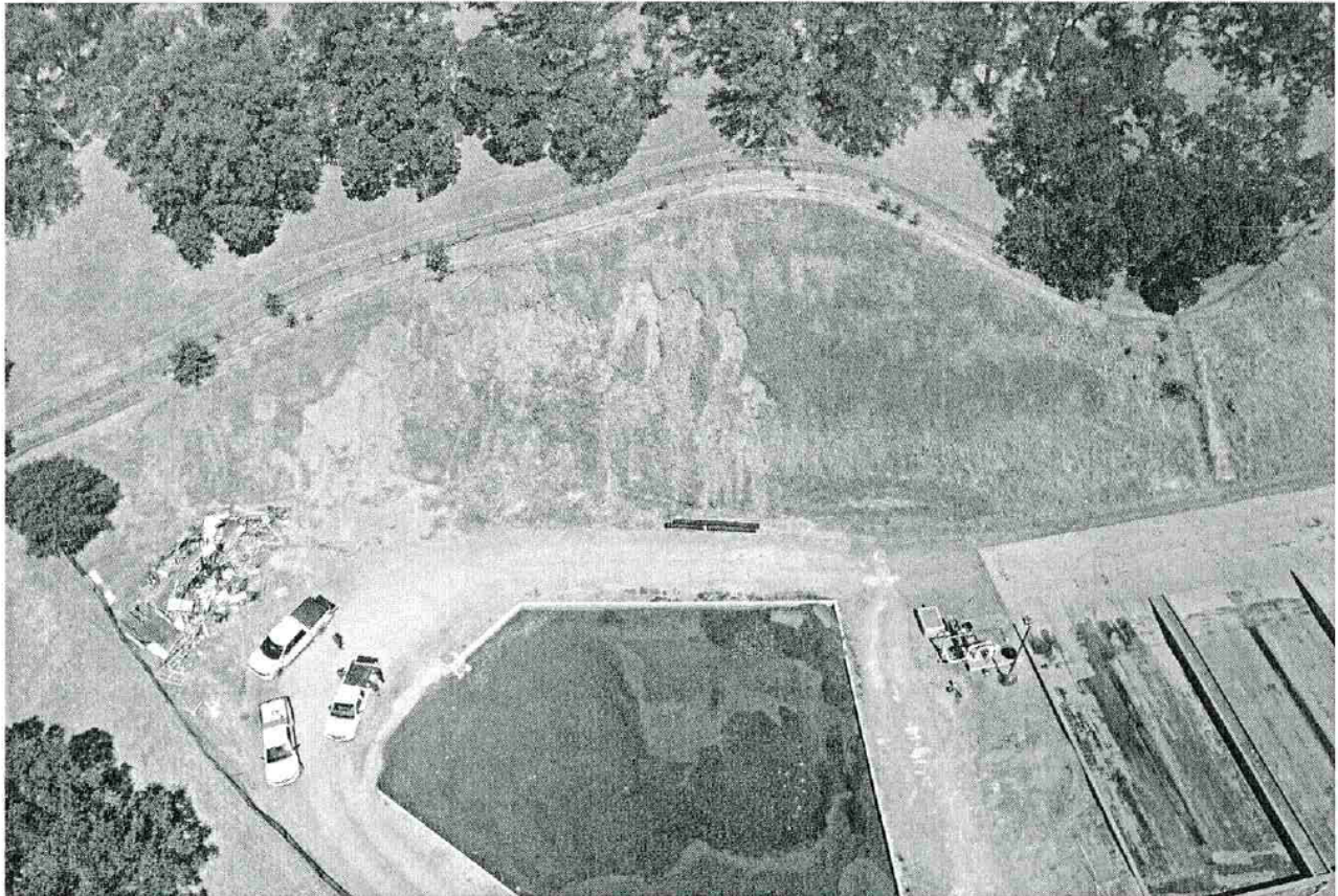
Figure 1: Aerial drone derived photo of the site (22 July, 2025)
