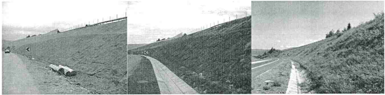
Figure 3: Example of a pinned mesh slope (during installation, immediately after revegetation, and with developed mature grass).
